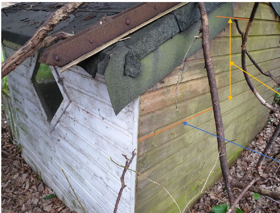
This picture has the laser level line from the front door threshold of 29 Westcote Road projected onto the rear of the summer house showing that it is ~0.5m below the 18/16 Parkside Road fence line.
